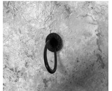
**Step 3:** Run a bead of 100% silicone caulk around the tube on the back of the control. Make sure there is enough to fill any grout lines and that the silicone is far enough from the edges to remain hidden after mounting to the wall. **Note-** *If using optional trim ring (K2 control only), install trim ring over the back of control first.*
